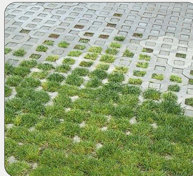
Erosion/compaction control unit (precast/plastic) infilled with recycled aggregate and soil.
