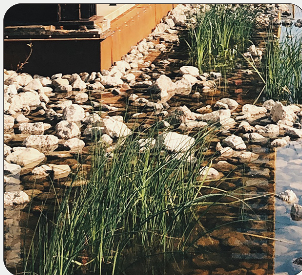
Crushed and tumbled recycled aggregates 20mm - 300mm DIA to creekline and garden beds.
