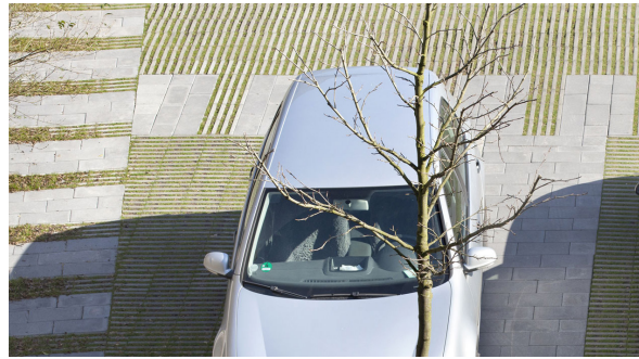
Permeable car parking spaces with integrated planting
