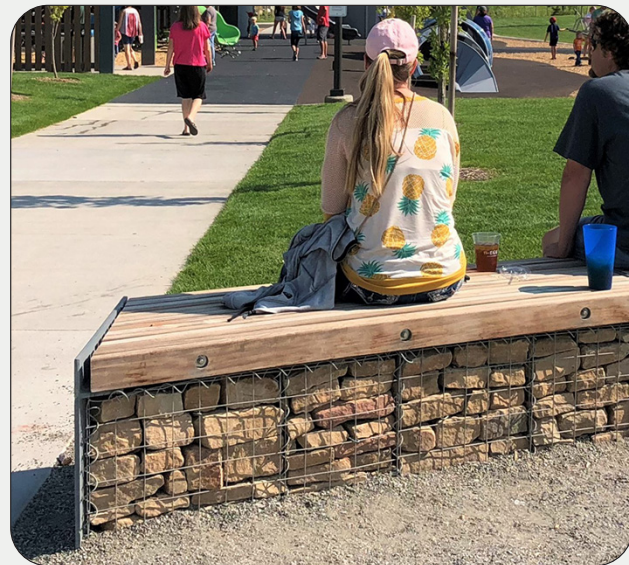
Gabion walling fitted with supporting steel structures to provide seating finishes/materials.
