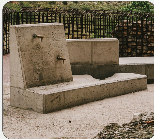
Surplus concrete insitu forms used as seating plinths. Finishes could include adhoc boarding and varying concrete types layered.
