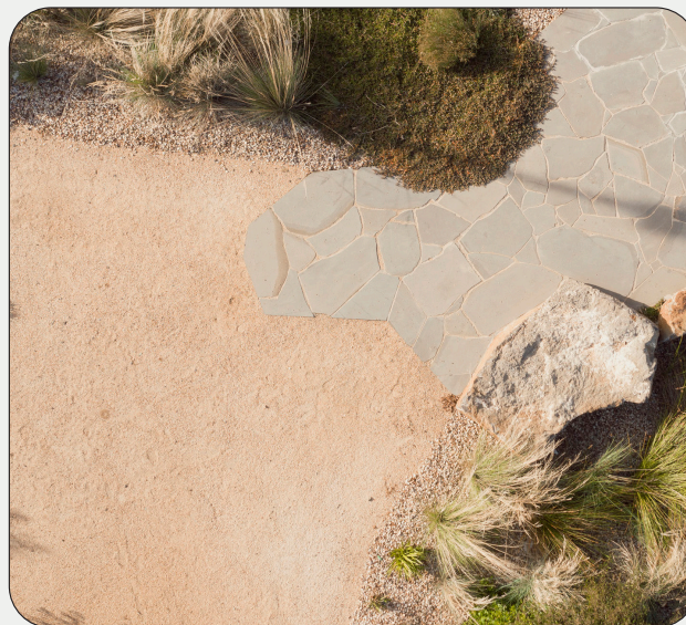
Crushed recycled aggregate path. Aggregate to include recycled concrete, tiles, and glass or similar.
