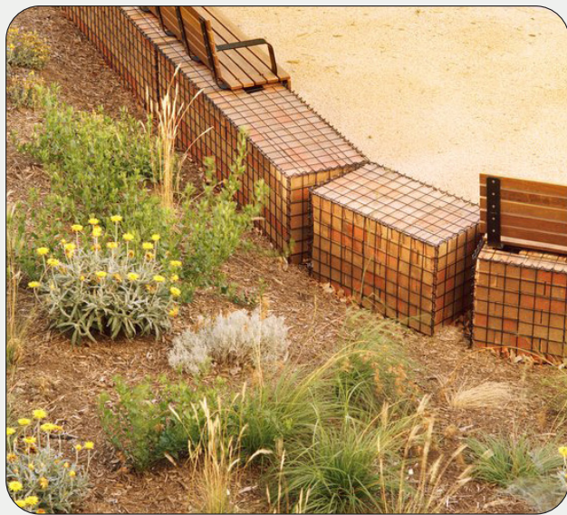
Gabion cages with compliant timber backrests.
