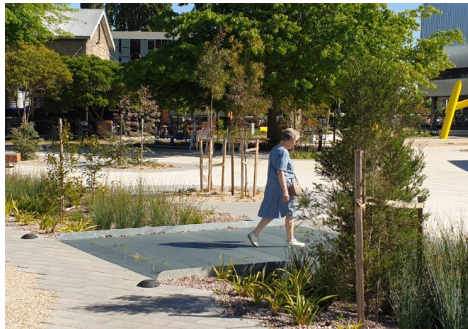
Swale as linear blue/green treatment system
