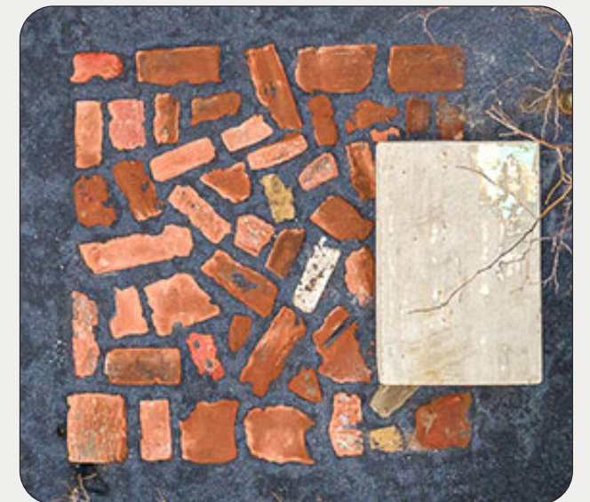
Mosaic of random recycled unit pavers (recycled pavers, tiles, concrete slabs and aggregates).
