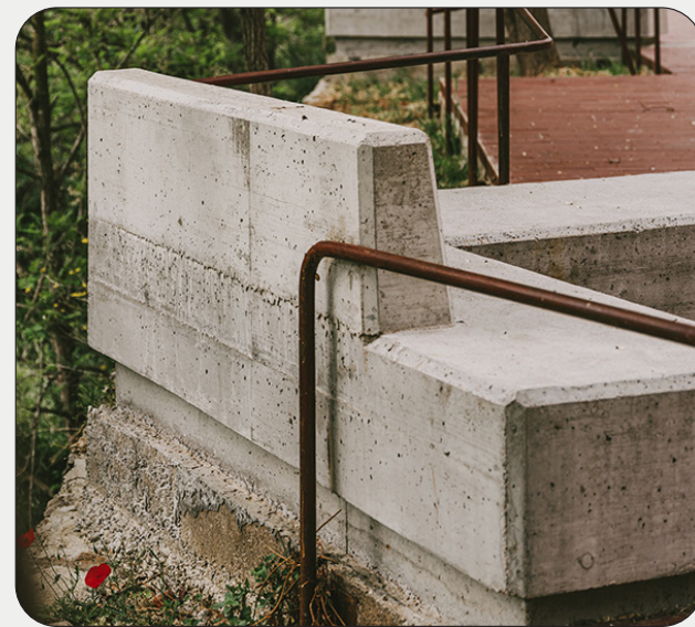
Recycled metal pipes such as fire sprinkler systems used as handrails and balustrades.
