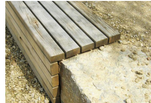
Gabion cages clad with timber for pleasant seating nooks
